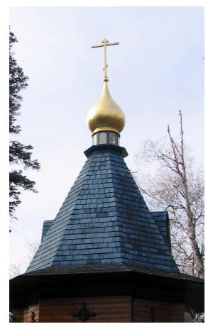
The main cupola from Saint Sergius Chapel blew off in a winter storm. Inspection revealed that water had seeped in and rotted the base where it was bolted onto the roof. This cupola is now sitting behind the Church shop and available for inspection.
